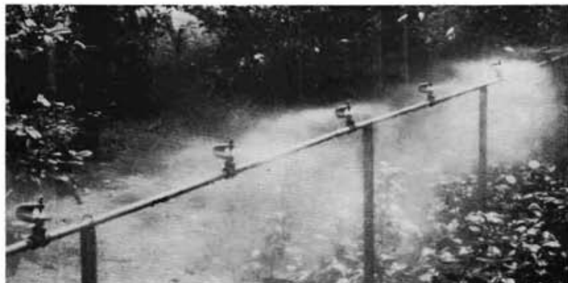
Typical Installation of Mister Bs in Series
