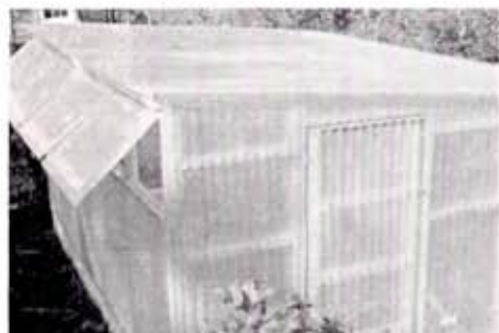
Above is an all corrugated fiberglass greenhouse, which can be built by average handyman. Note ventilation features.
