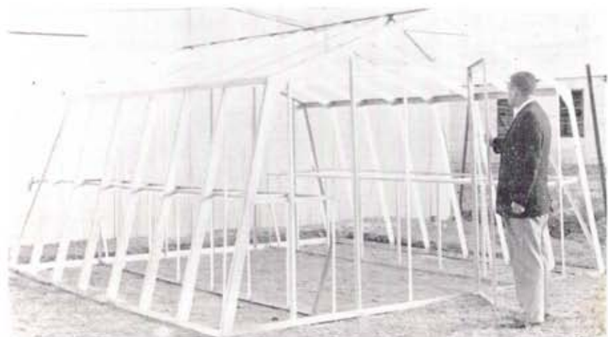
Here is metal frame-work for an all plastic greenhouse. Easy to erect and cover with polyethylene plastic. Can be extended in units of four feet.
