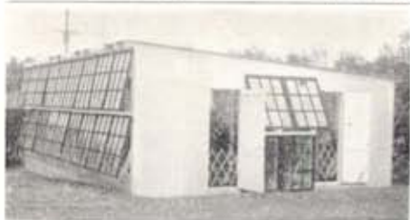
Another example of combination fiberglass and glass using second-hand window-frames. Note top and bottom ventilation on all sides.
