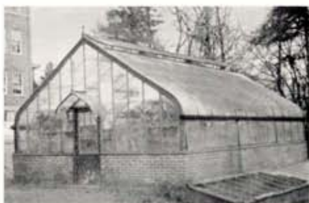
Seen above is a prefabricated all-glass house with metal framework, relatively free of upkeep except for broken glasses. Many of newer models have better ventilation for Camellias.
